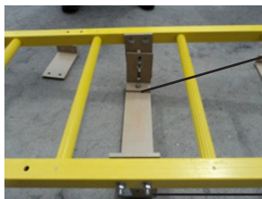
Support bracket bolted to ladder rails
