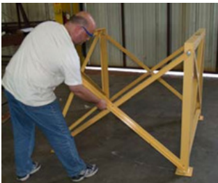
Assemble Side Angle Braces
